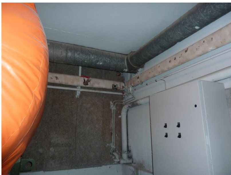
X1/ PRELEVEMENT CALORIFUGEAGE CHAUFFERIE LT 29
